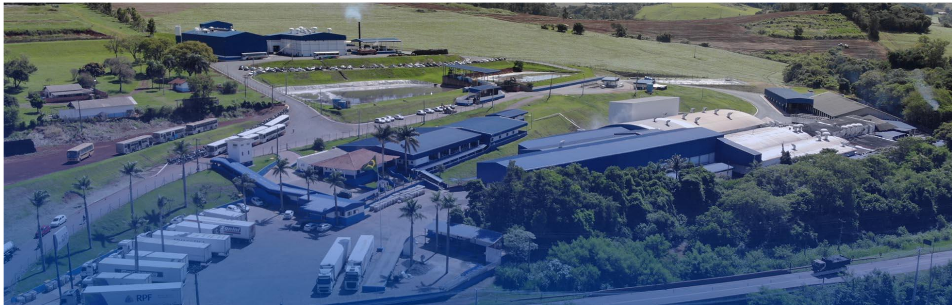
Complexo Industrial de Ibiporã/PR
